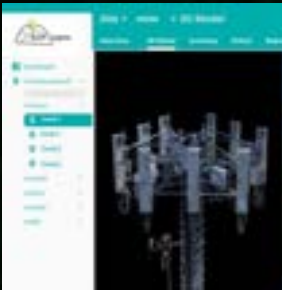
Cell Tower Inspection (LTC 4 )
