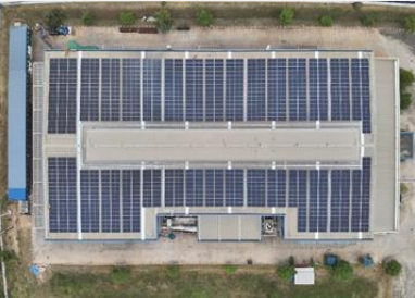
SFT2 : 0.54 MWp New installation 2024
